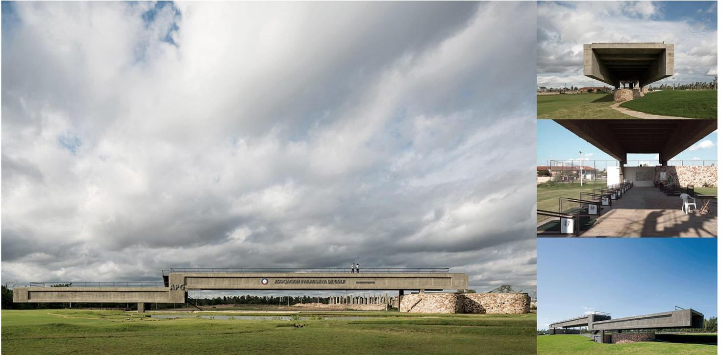
The roof of the APG Paraguay building is designed to be used as a golf driving. Due to this, the cover is flat with a 2.5m-high terrace.
